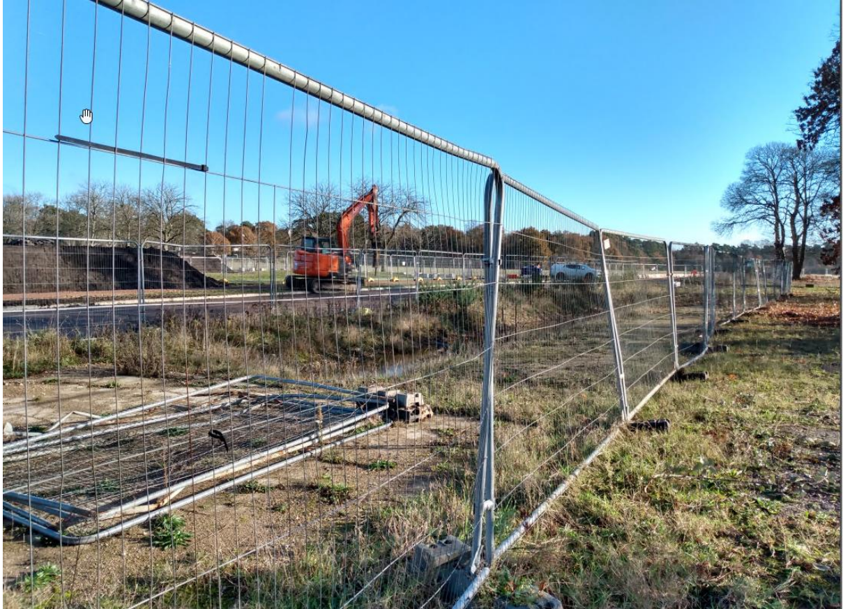
Recent site photo – showing redevelopment at rear of site
